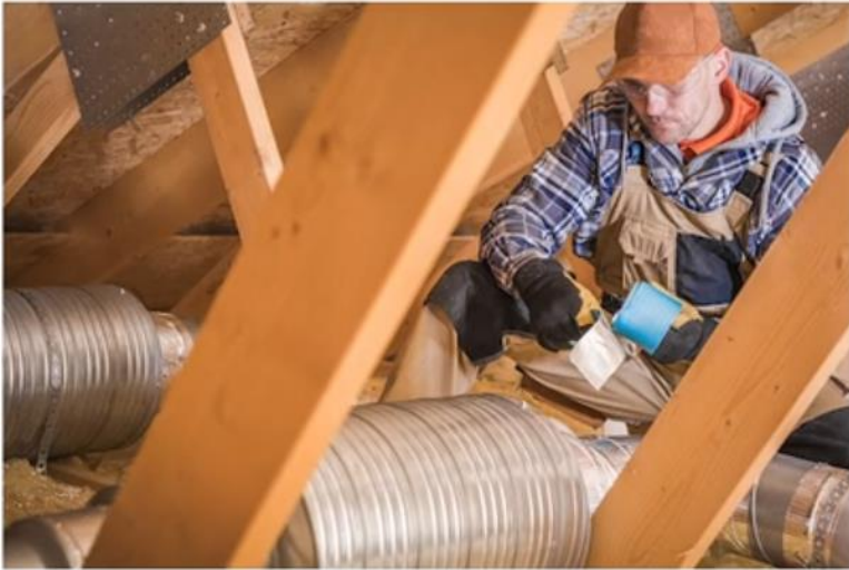
Duct Sealing
